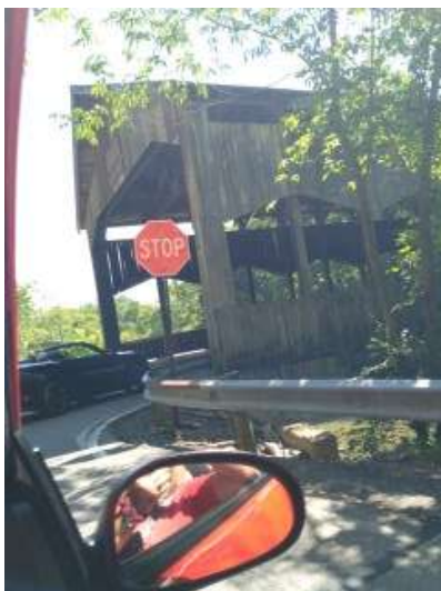
Covered bridge along the pony trail.
